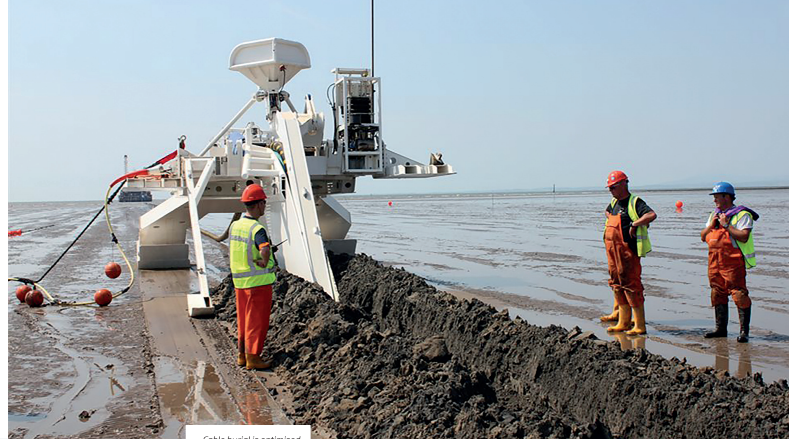
Cable burial is optimised for site conditions.
