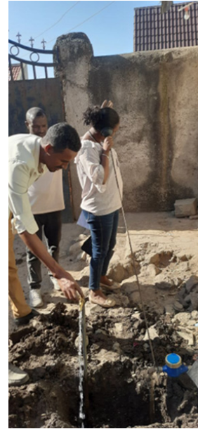
Figure 5: On-site coaching on listening rod for leak detection utilization
