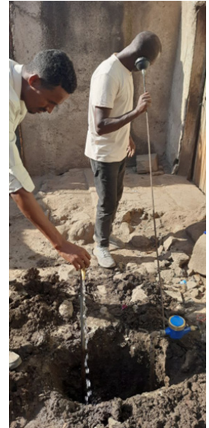
Figure 5: On-site coaching on listening rod for leak detection utilization
