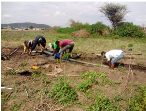
Figure 3: Bulk water meter installation at the inlet and outlet of the DMA
