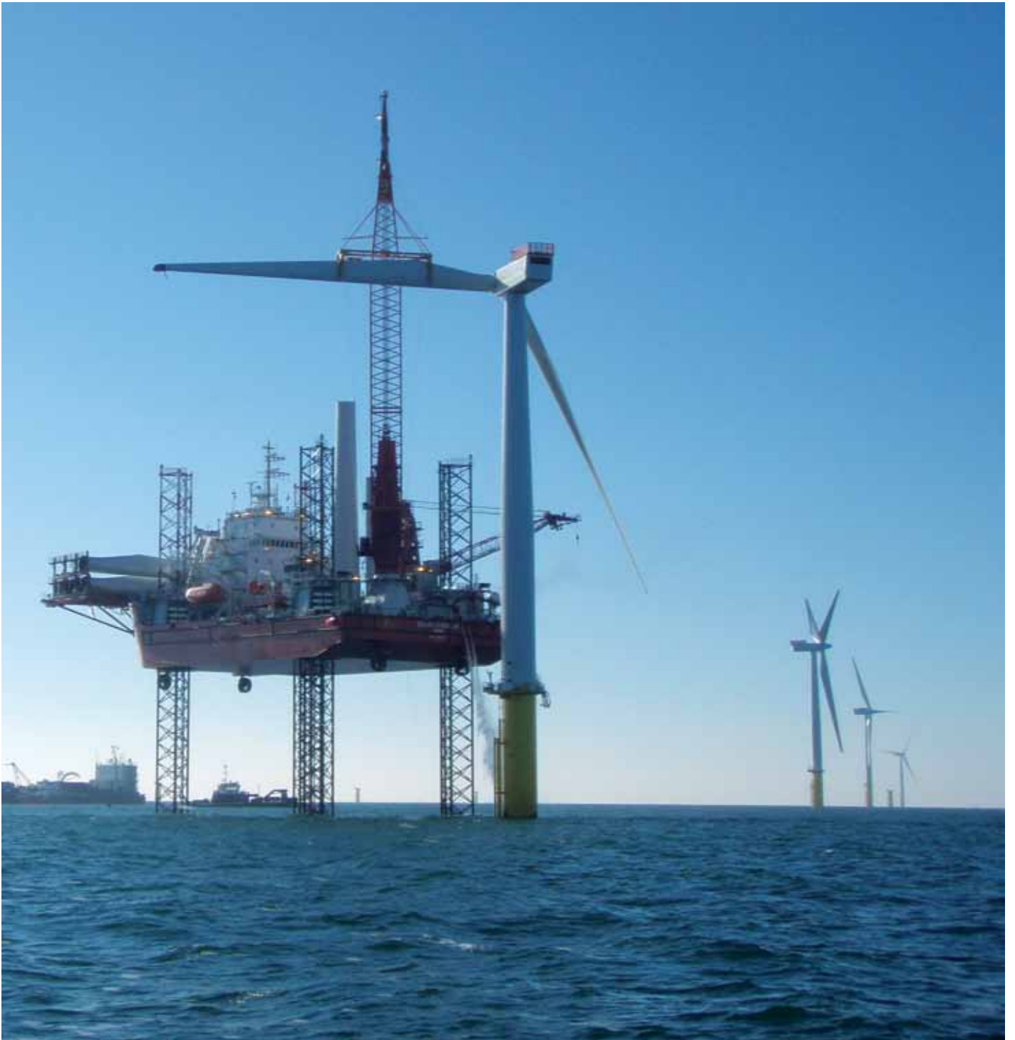
Walney Offshore Windfarm I & II
